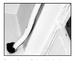
If a pencil eraser fits in a hole, there's room for a mouse. You can use steel wool to plug up a hole (like the one around the conduit in this picture) so mice can't squeeze through.
